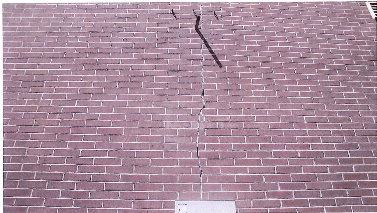
East Elevation – Veneer Crack, View #2
