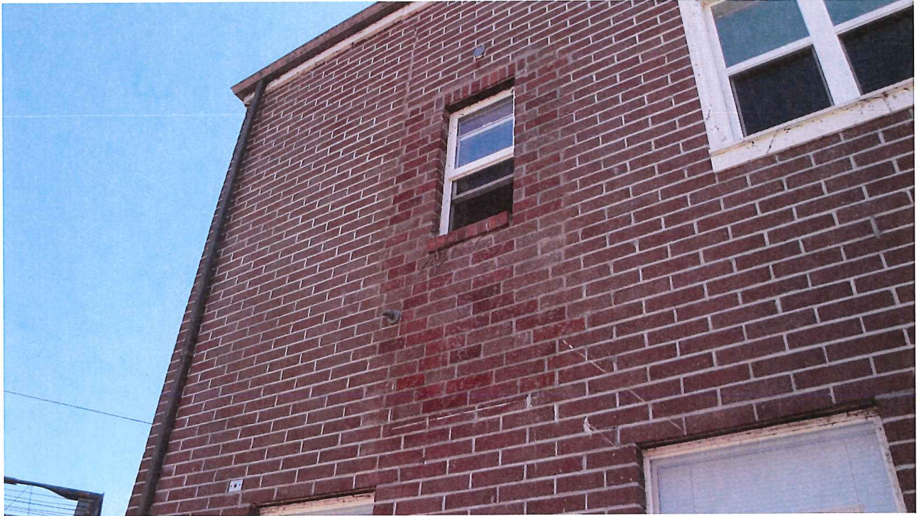
West Elevation – Large Area Veneer Replacement
