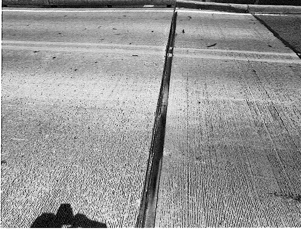
7) East Expansion Joint, Looking North
