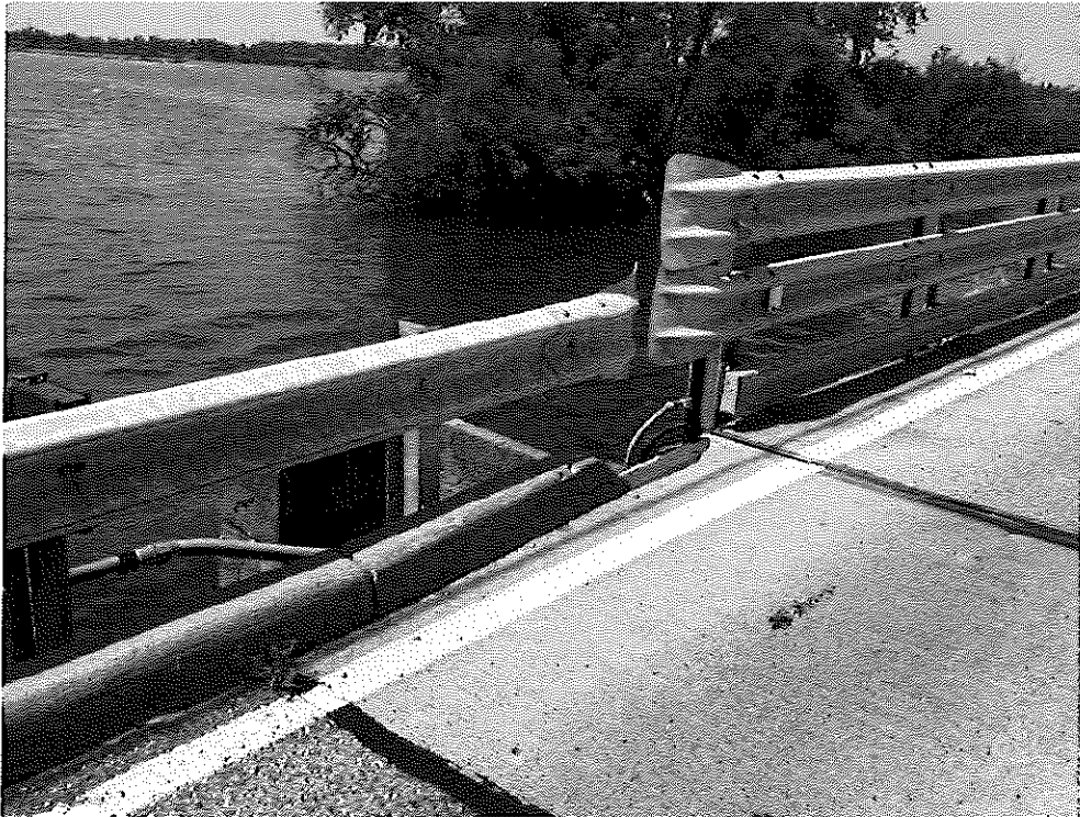
10) Southeast Approach Quadrant
