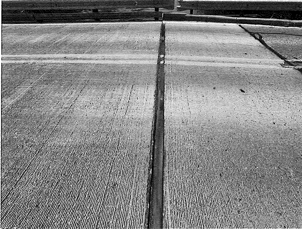
8) West Expansion Joint, Looking South
