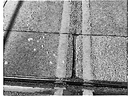
Photo S-04 [Span 4] Concrete spalling at joint between Span 3 and 4, looking west
