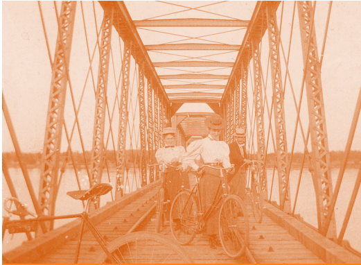
BICYCLISTS ON THE FREE BRIDGE
