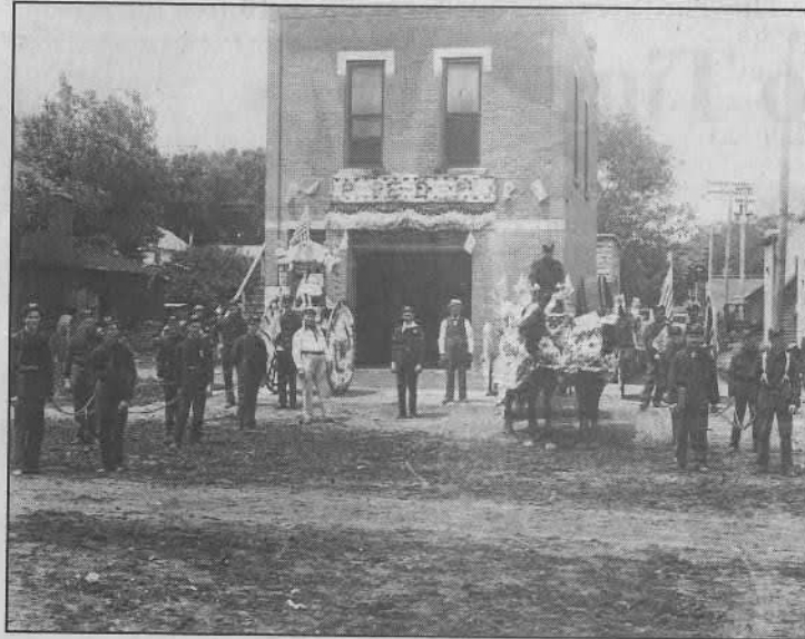
Early day Concordia fire laddies were all dressed up to have their picture taken. The doughty firemen had decked their hose carts with bunting and decorated the city hall/fire department building which then stood on the site now occupied by the post office. Photo taken July 4, 1899.
