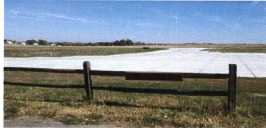
Typical permanent fencing at Blosser Municipal Airport that does not provide adequate access control to sensitive areas of the Airport
