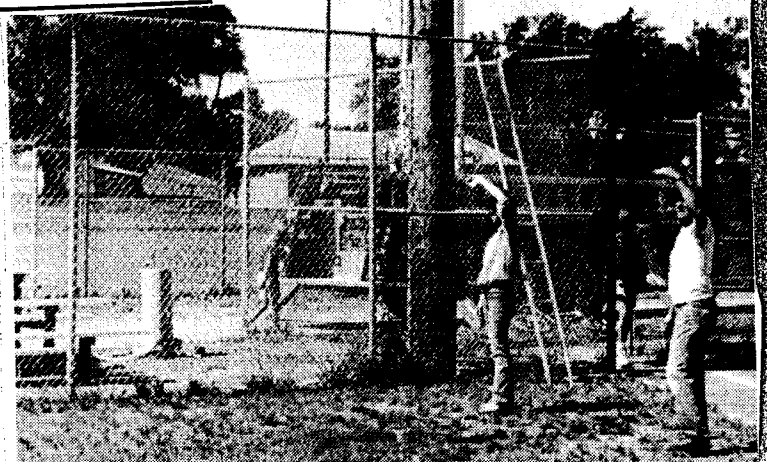
SAFETY NETTING —Safety netting was being installed behind three of the backstops at the Concordia Sports Complex over the weekend. Volunteers were busy attempting to
