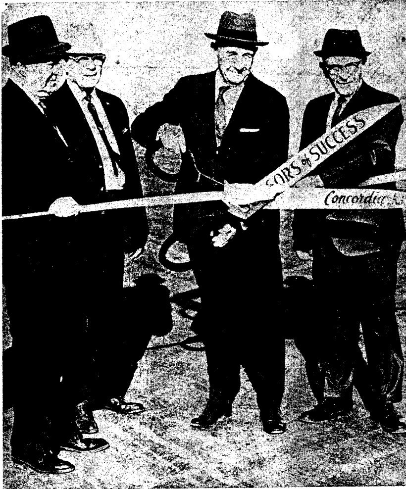
AIRPORT OFFICIALLY OPENED —Senator Frank Carlson cut the ribbons yesterday afternoon to officially open the new hard surface runway at Blosser Municipal Airport in Concordia. Others in the picture are (left to right) J. R. Hall, general contractor; Charles Blosser, Carlson and Mayor Harry Gotschall. (Blade-Empire Photo and Scan-a-graving.)
