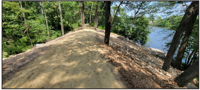
The old wooden footbridge in the Fontana Woodland was replaced with a rock crossing.
